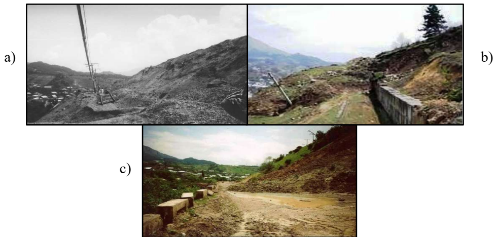
Fig. 2. The railway destroyed by a landslide - a); blocked by climb down masses the railway track - b); the bypass road - c).
