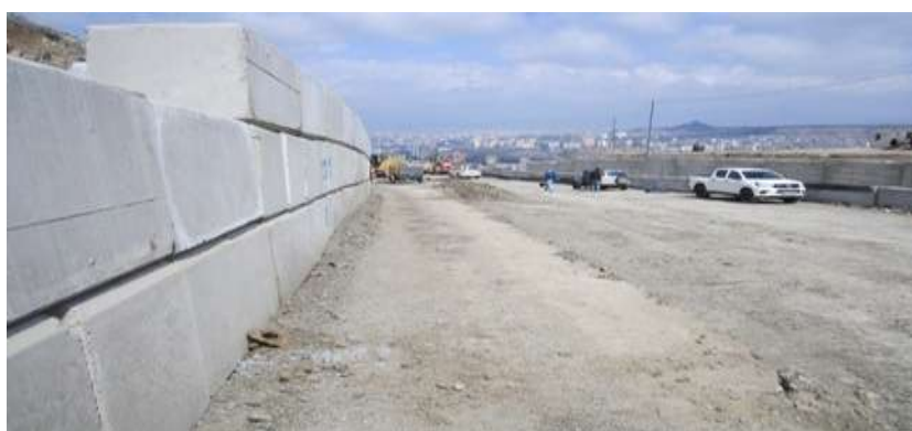
Fig.3. Georadar work area along the concrete wall
