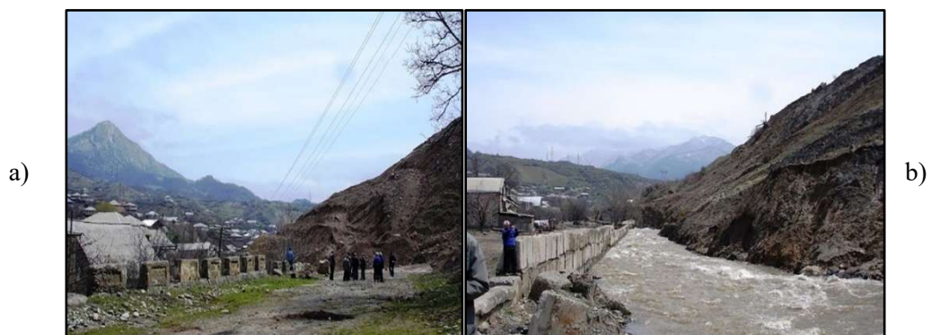
Fig. 4. A bypass road blocked by a landslide - a); landslide masses that collapsed into the riverbed of the Aghstev river - b).
