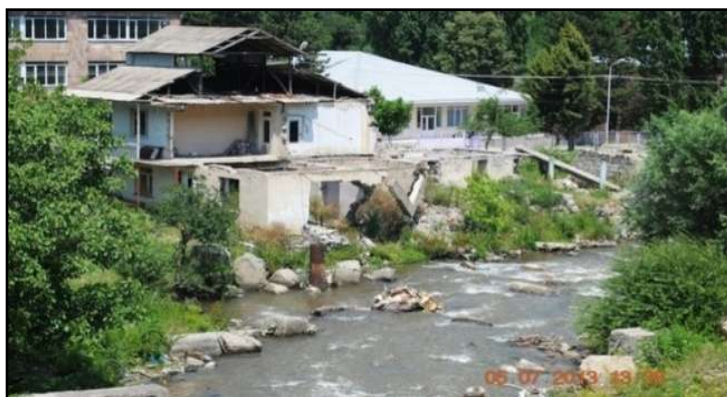
Fig. 5. Destroyed buildings on the left bank of the Aghstev river (05.07.2013).
