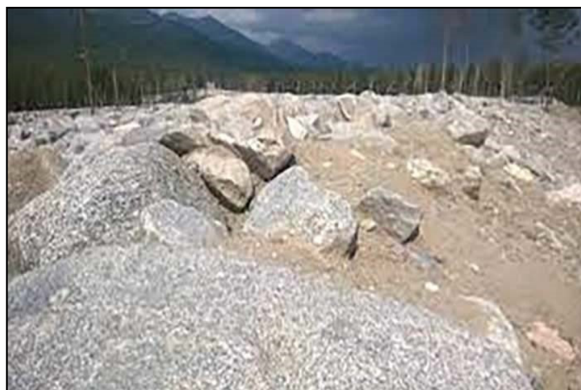
Fig. 5. Mud-stone mass that blocked the railway tracks on the Alaverdi-Akhtala stretch
